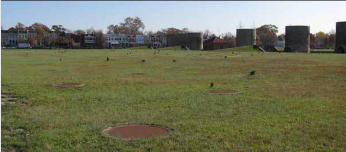
View of rows of manholes on top of filter beds.
