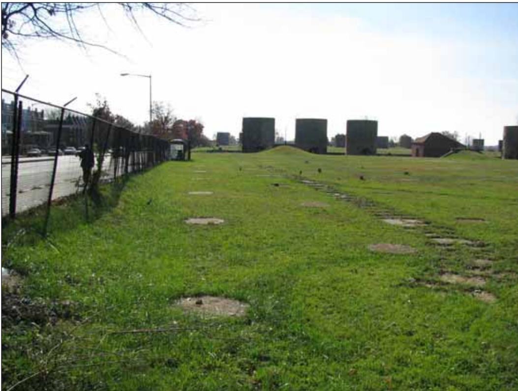
View of east side of site, looking south from northeast corner
