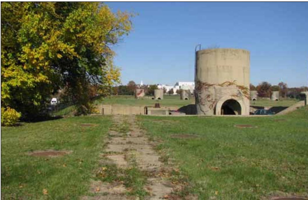
1. View looking north from the western leg of the path, views north point to the tower of the historic Forwood Building. (1906), which contributes to the Armed Forces Retirement Home-Washington Historic District, which is listed in the National Register of Historic Places and in the DC Inventory of Historic Sites.
