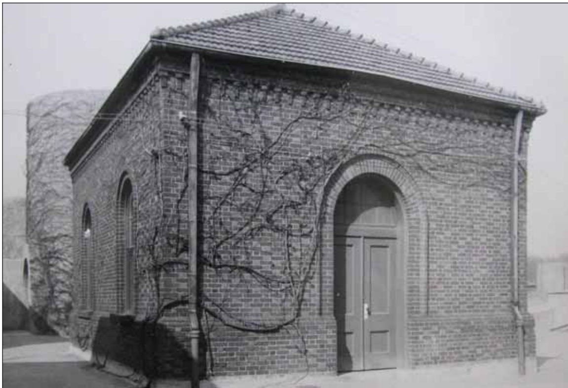
View of Regulator House, 1944
