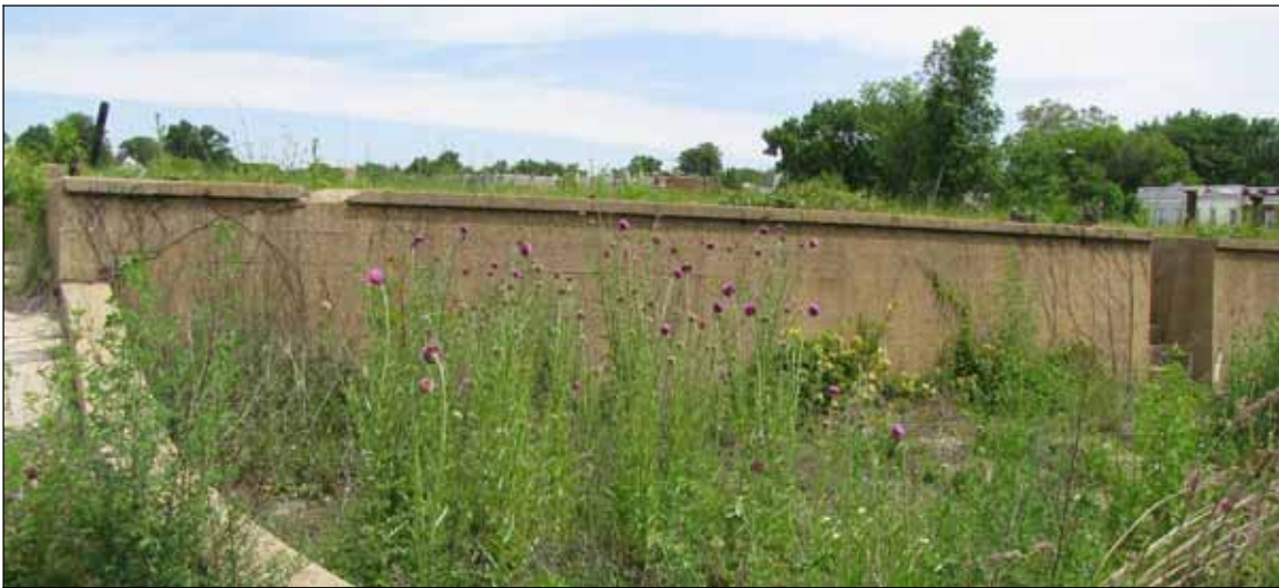
Typical wall of service court
