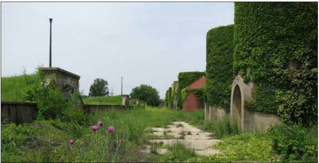
Existing conditions of Service Court No. 3 looking west (spring), EHT Tracerics, Inc., 2008
