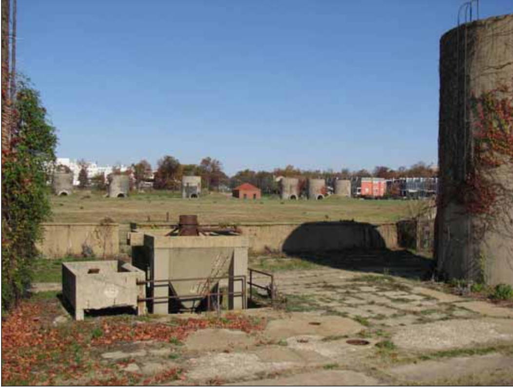
6. View from southern service court looking north to the northern service court
