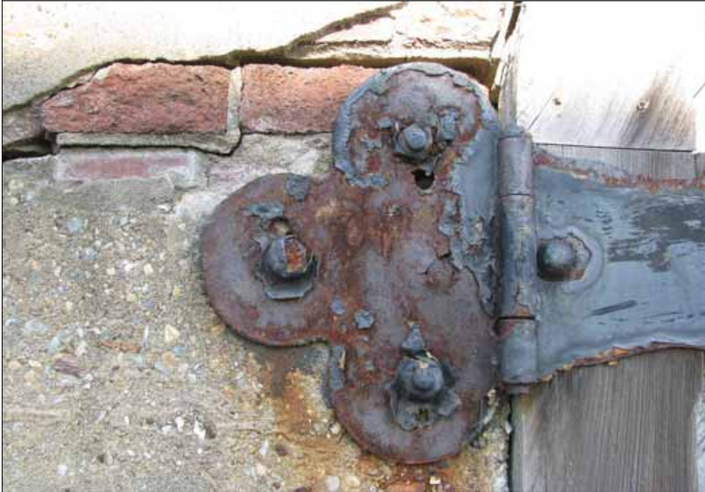
Typical iron hardware on filter bed portal
