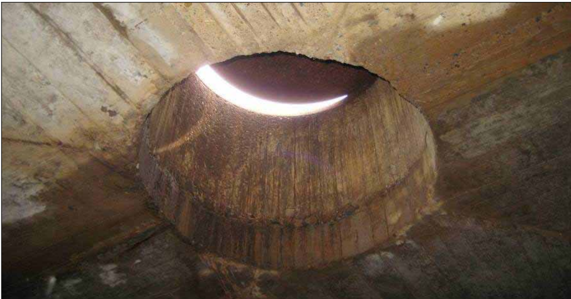
View of manhole from interior of filter bed
