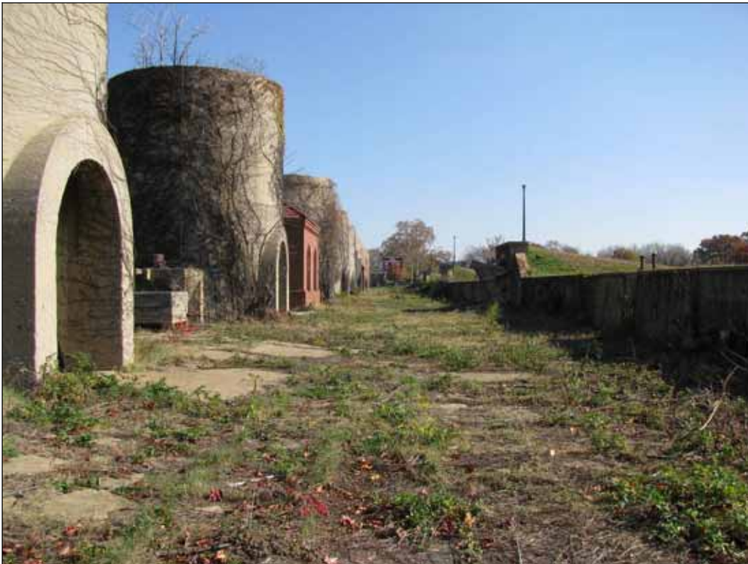
5. View looking east from west side of northern service court
