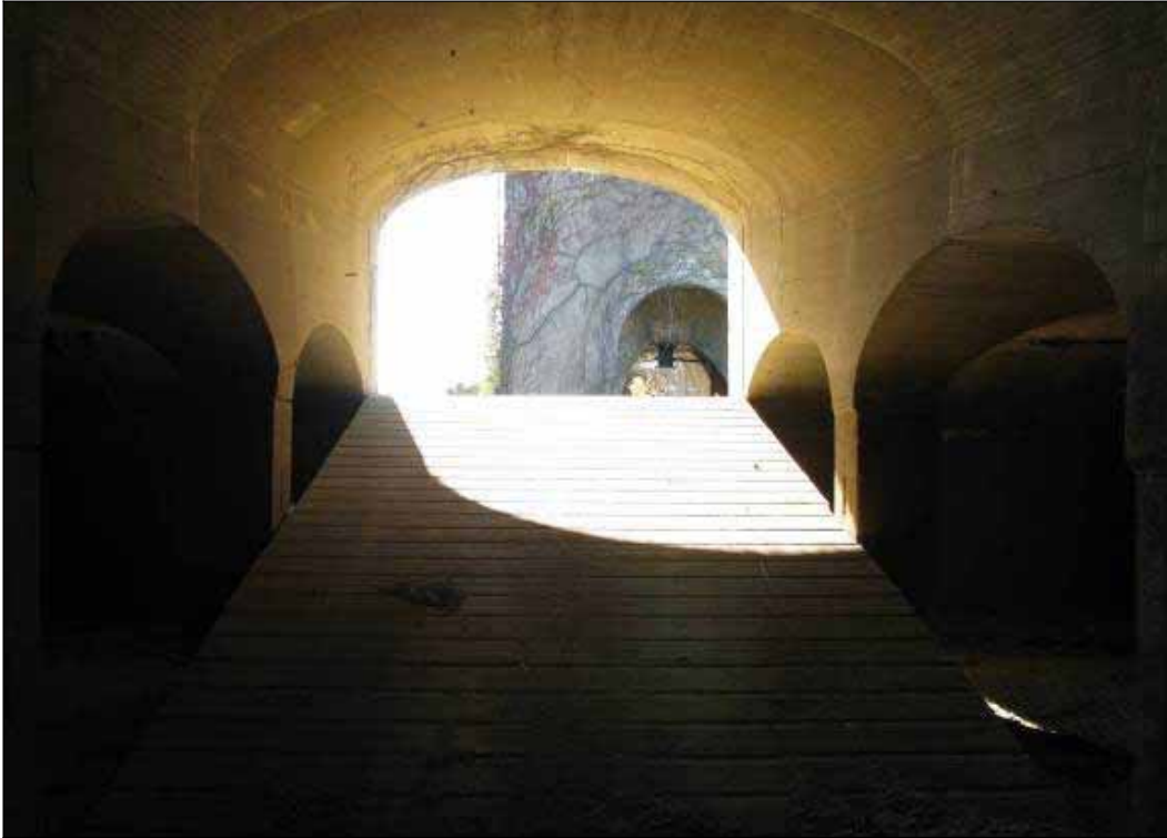
Ramp from filter bed to service court
