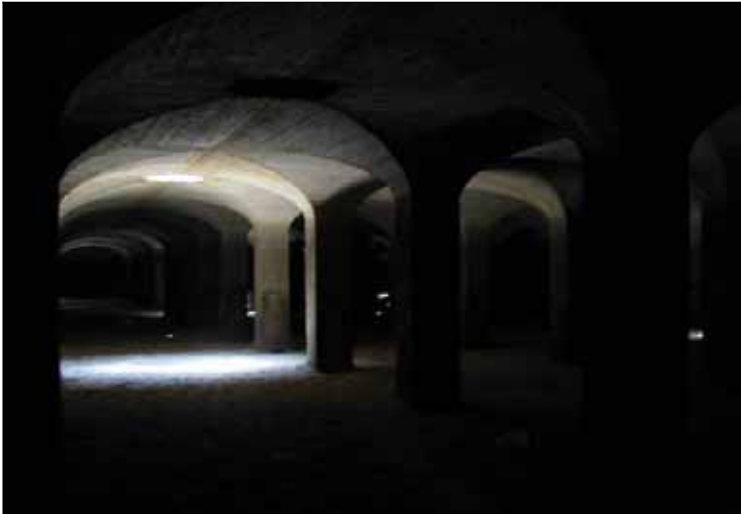
Typical interior of filter bed
