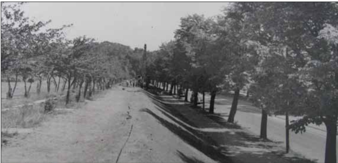
Image of perimeter plantings during trench work, July 1946
