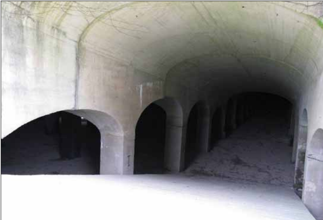
Ramp from service court to filter bed
