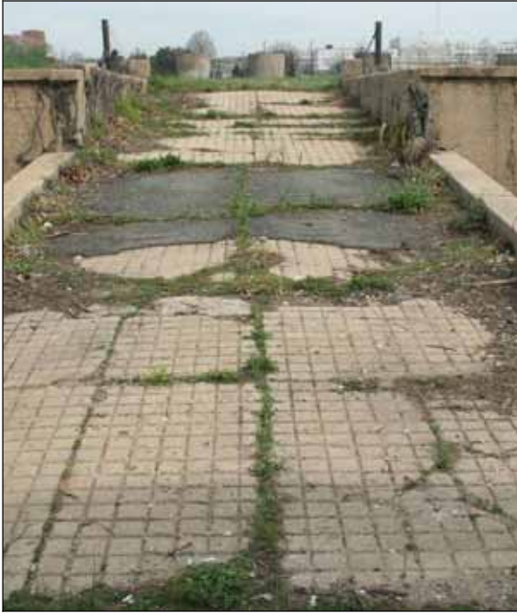
Ramp showing grid pattern in concrete
