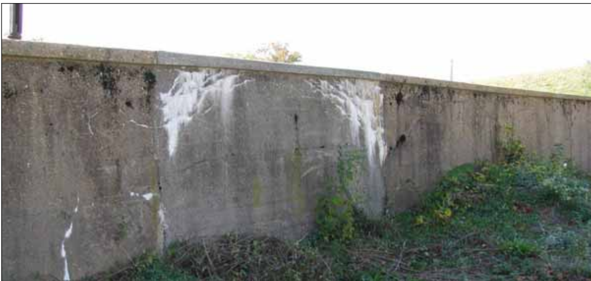
Infill of wall of service court where ramp was demolished
