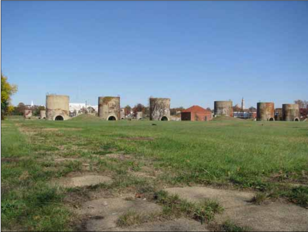
2. View looking northeast from southwest corner of site (intersection of Channing Street and First Street)
