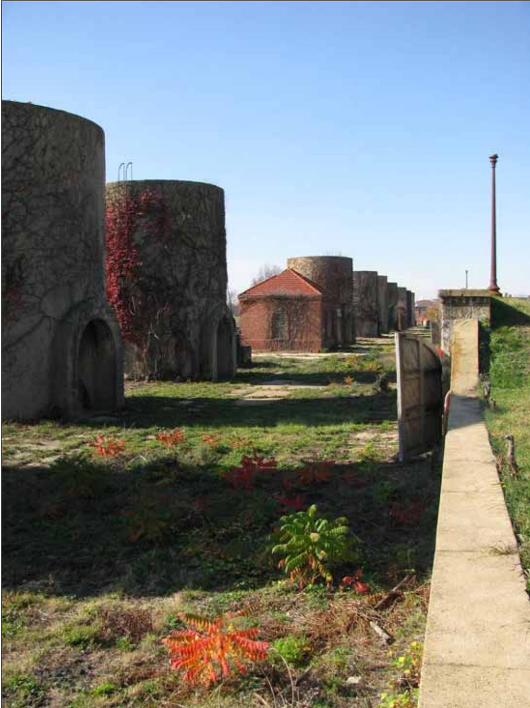
7. View looking west from east side of southern service court
